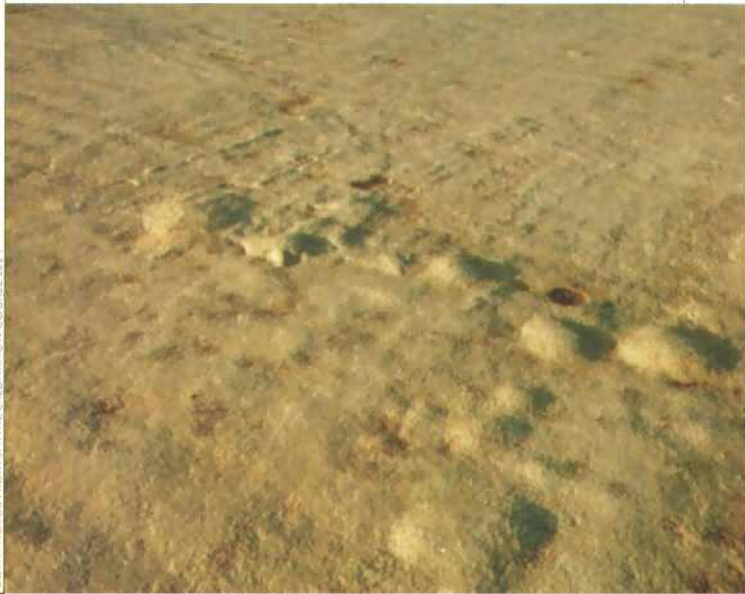
Above: Blisters on a SPF roof are typically caused by thin foam passes and/or moisture or contaminants on substrate. Left: Mechanical damage typically does not cause leaks in SPF roofing systems and can be repaired with a compatible sealant.
