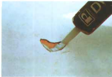
Above: Blisters on a SPF roof are typically caused by thin foam passes and/or moisture or contaminants on substrate. Left: Mechanical damage typically does not cause leaks in SPF roofing systems and can be repaired with a compatible sealant.
